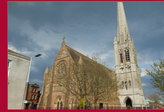
03. ST WALBURGE'S CHURCH Built in the mid 19th century by the Gothic revival architect Joseph Hansom and is famous as having the tallest spire of any parish church in England. 0.3 miles | 7 mins | 2 mins
